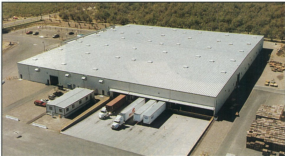
Outside of this 105,000 sq. ft. warehouse is Escalon Premier Brands' 1,000 sq. ft. human resources department office
