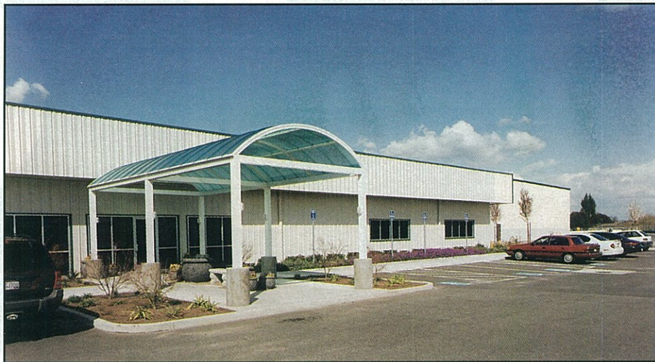
Span Construction added this fiberglass canopy to emphasize the entrance of the corporate office.
