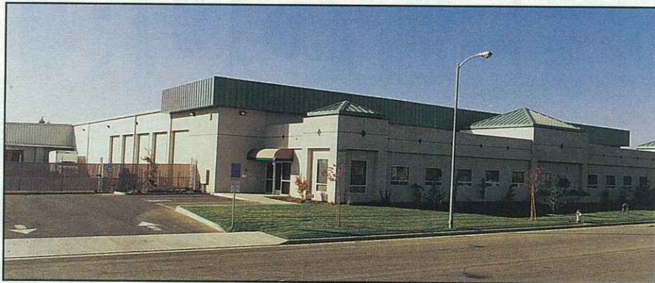
Span Construction still abides by the same principles that were instilled when it was founded. This is evident by the many projects the Madera, CA-based company, now in its 20th year of operation, has completed recently including this 30,000 sq. ft. MEPCO building in Fresno, CA (above).
