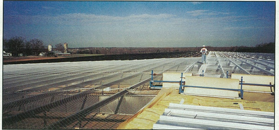
A pair of Span projects shown under construction: Salt Lake City (UT) Recycling Center (left) and CFG-Cardinal Float Glass Plant (above) in Mooresville, NC. As evidence of Span's company-wide concern for safety, netting helps to protect workers.
