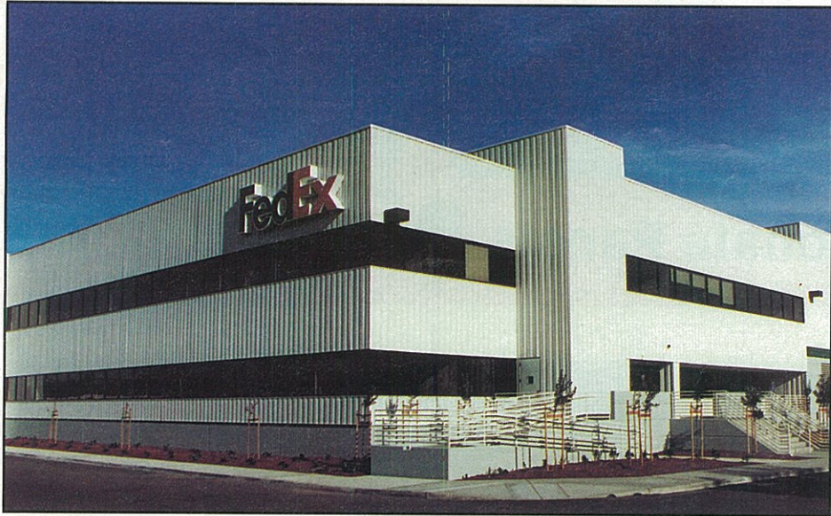
This Federal Express project by Span is located in Oakland, CA, and measures 228,00 sq. ft.
