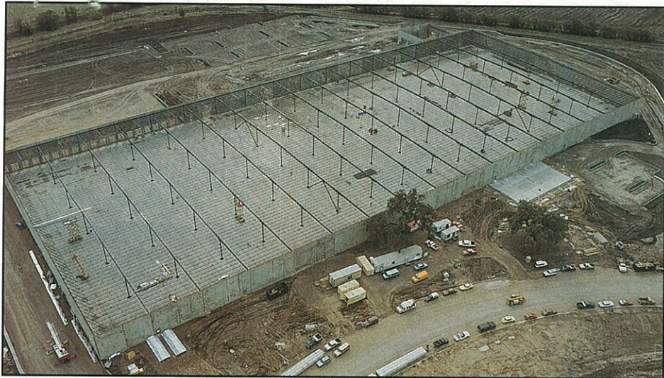
The 306,000 sq. ft. Noll Manufacturing facility in Stockton, CA, features full height concrete walls and a standing seam roof. The photo to the left shows a full aerial view of the structure. To the right is a closer view of the inside of the building under construction.
