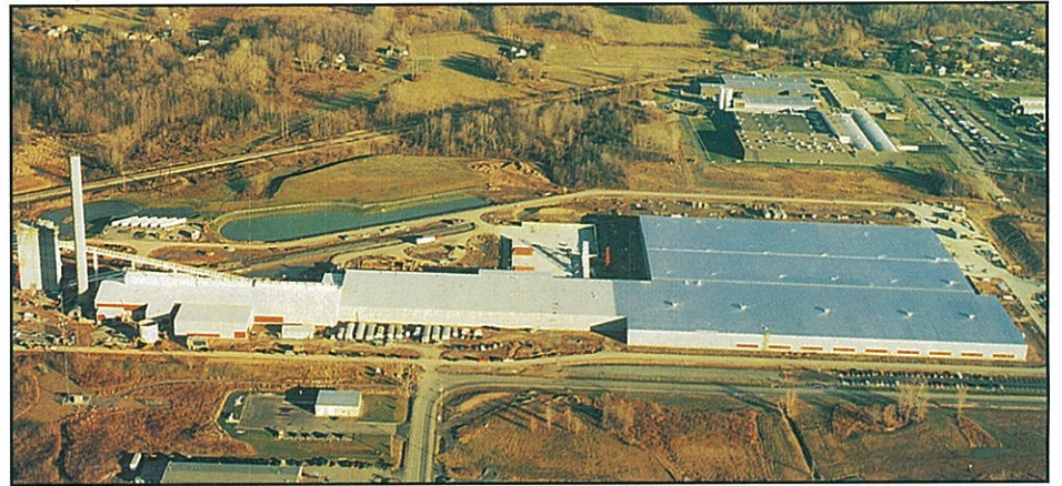
Span Construction & Engineering used pre-engineered building systems from VP Buildings for the mammoth Guardian Industries facility in Geneva, NY.
