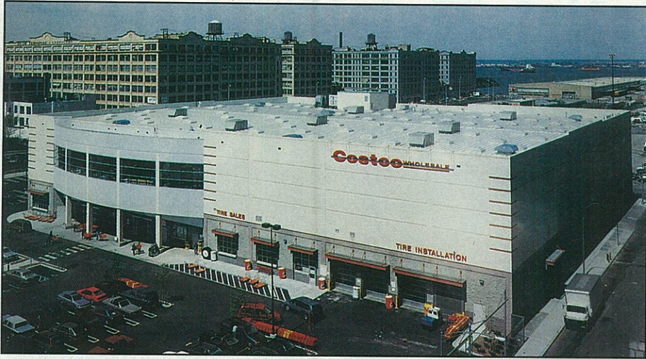
Costco Wholesale, Brooklyn, NY, is one of many projects Span has completed for Costco.
