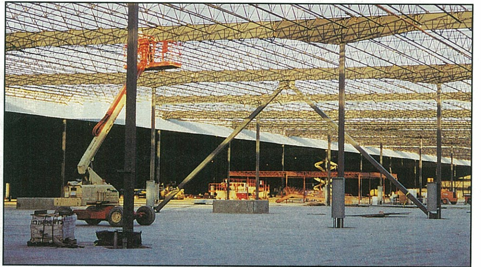
The 306,000 sq. ft. Noll Manufacturing facility in Stockton, CA, features full height concrete walls and a standing seam roof. The photo to the left shows a full aerial view of the structure. To the right is a closer view of the inside of the building under construction.
