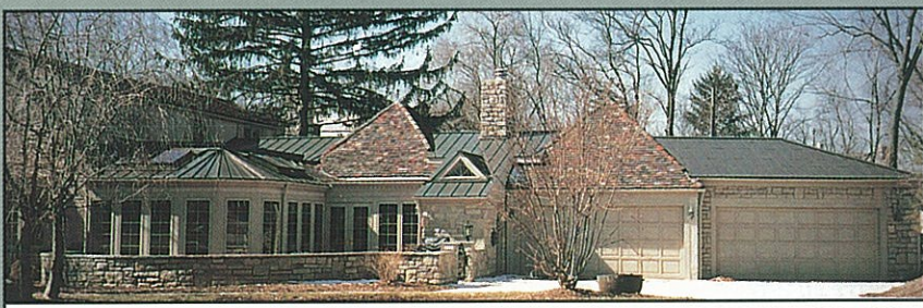
EIGHTH PLACE CUNNINGHAM RESIDENCE - UPPER ARLINGTON, OH Roofing Wholesale, Columbus, OH
