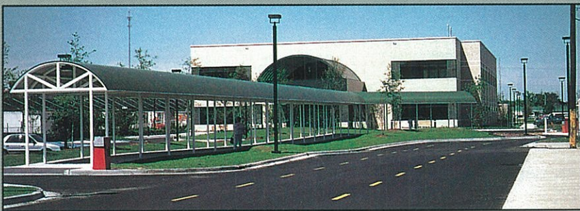
SIXTH PLACE OCHSNER DIALYSIS CENTER - NEW ORLEANS, LA Boes Iron Works, New Orleans, LA
