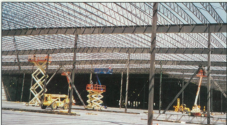
Using a Varco-Pruden truss system, construction begins on the Ball Glass Plant distribution warehouse (left) in Fairfield, CA. The impressive Ball Glass Plant project by Span measures 623,000 sq. ft. and is shown complete (right).
