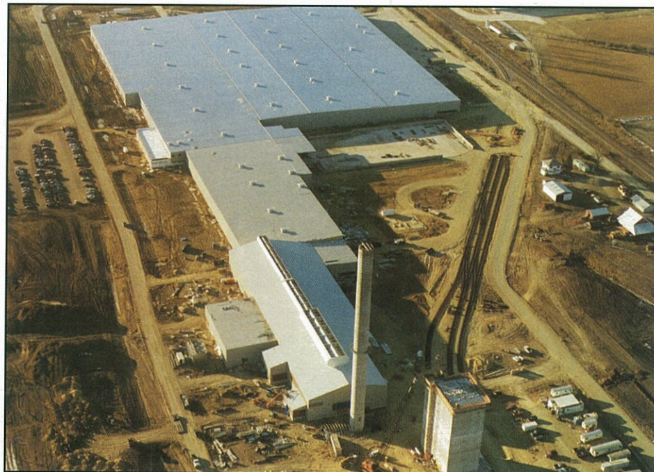
Span Construction & Engineering completed 65 projects in 1995, including this one for Guardian Industries in DeWitt, IA, featuring pre-engineered systems by Varco-Pruden Buildings.
