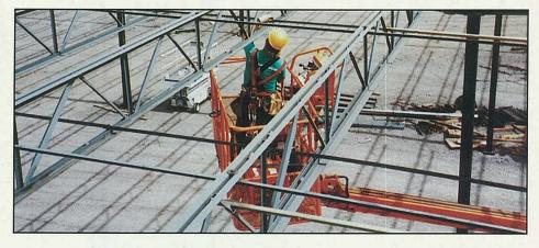
Span Construction requires vital, on-the-job safety training. Nylon safety netting is in place as an additional safety precaution on the roof of a 1994 PriceCostco project, Maui, HI, (shown at left). Proper safety reinforcements are shown while working on the roof of the Maui PriceCostco project, (above).
